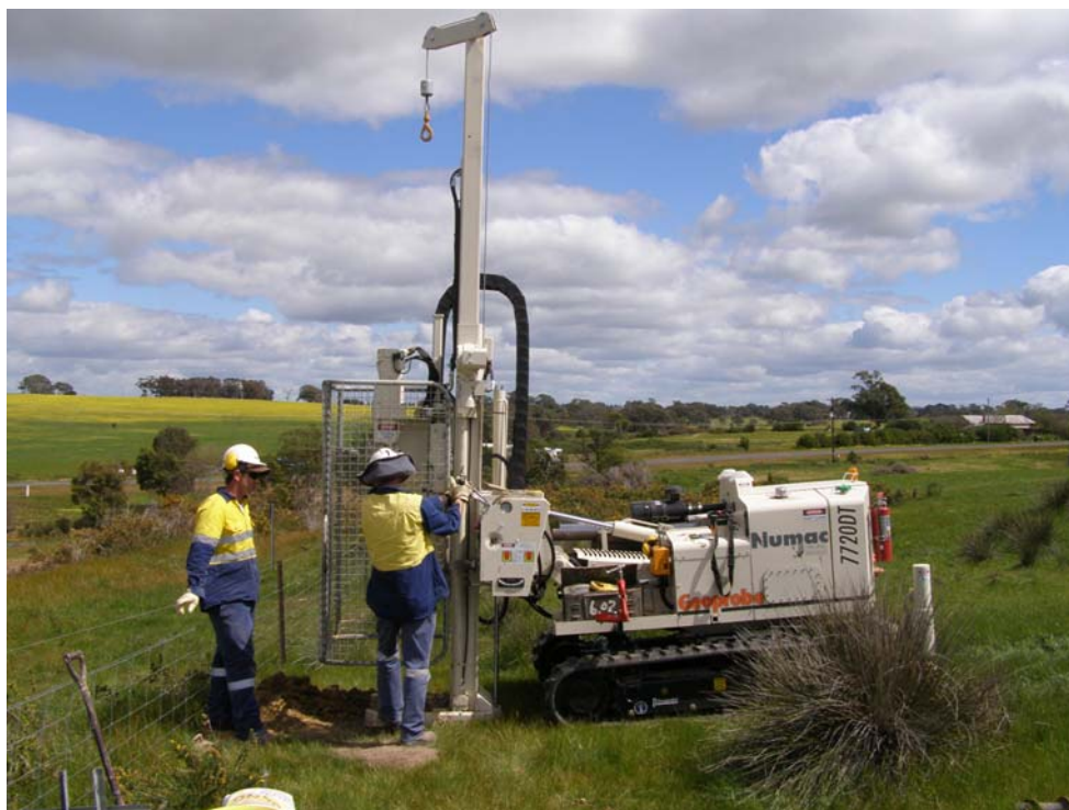
Figure 4-3 Piezometer construction using Geoprobe 7720DT.
