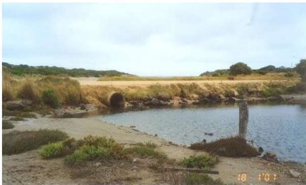
Original culvert connection through Point Impossible Road
