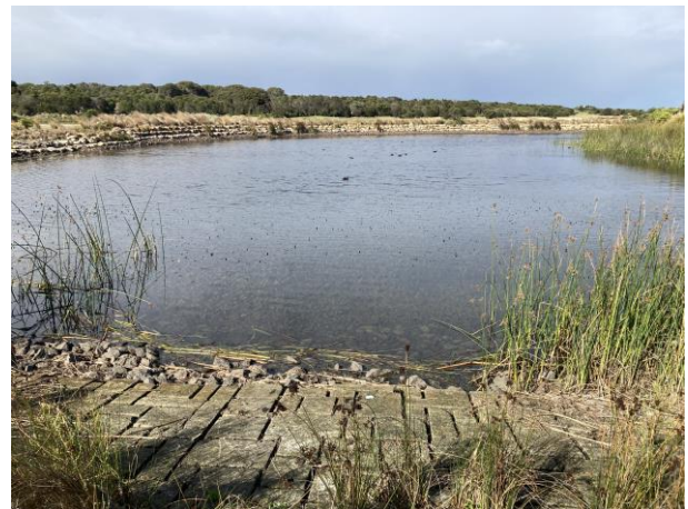
Stormwater pond adjacent to wetland
