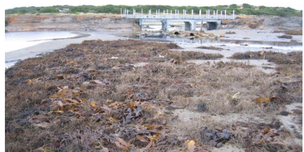
View of the new culverts during construction
