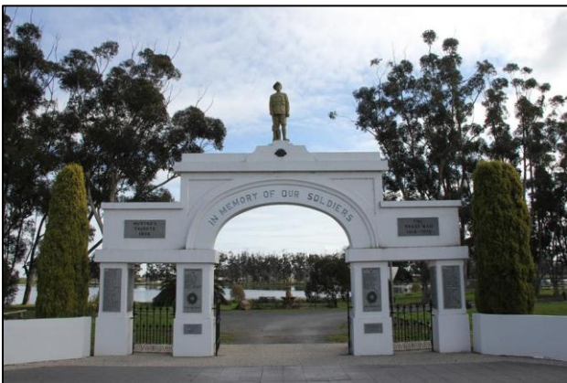
Figure 150 - Murtoa Memorial Gates, Lake Marma reserve
