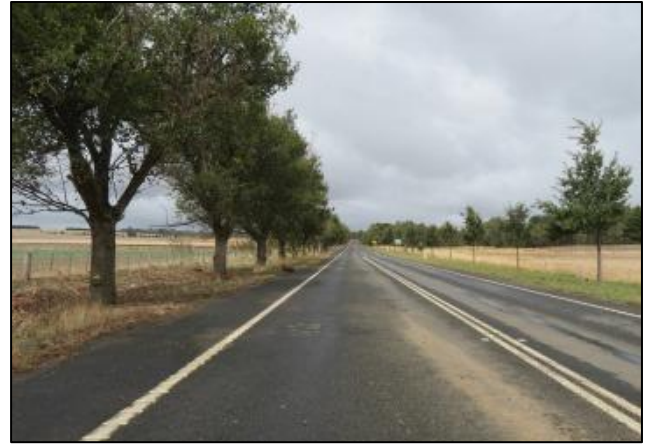
Figure 56 -Avenue looking south from Western Freeway roadworks
