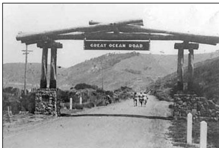
Figure 155 - Eastern View Memorial Arch, Great Ocean Road
